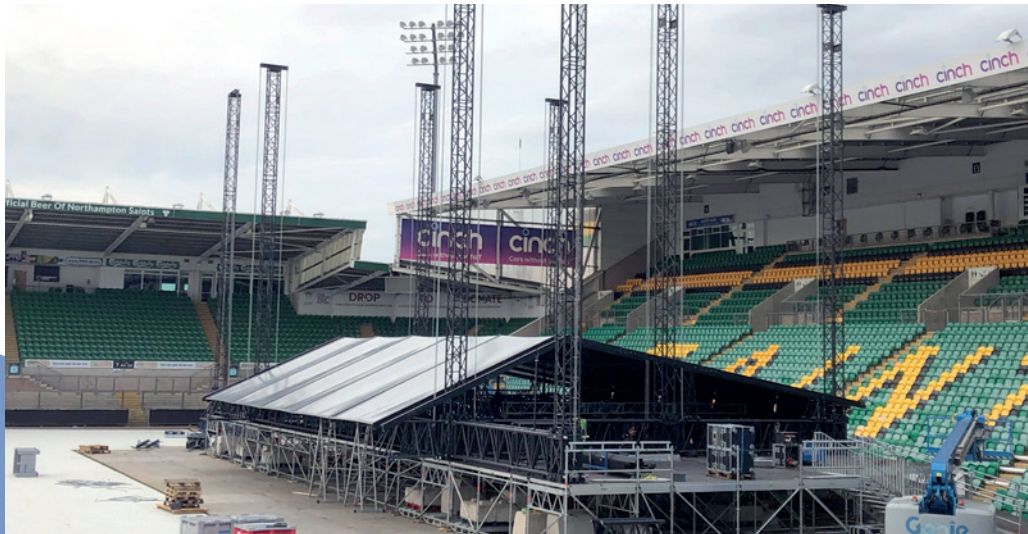
PR15 structure during construction
