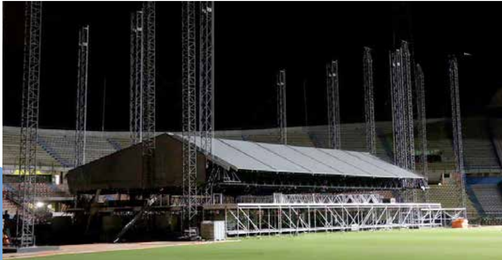
PR15 structure during construction
